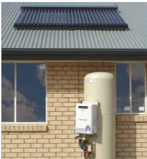
Figure 6: A typical residential solar hot water system with natural gas back up.
