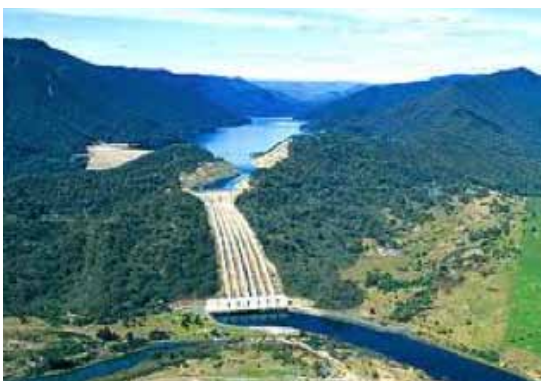
Figure 8: The Tumut 3 power station which forms part of the Snowy Mountains Hydro Electric Scheme.
