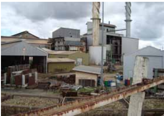
Figure 11: A Bundaberg Sugar steam generation plant.
