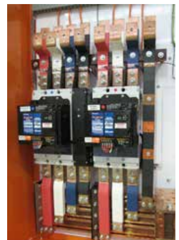
A typical circuit breaker based transfer switch, rated 1250A, with common load busbar assembly
